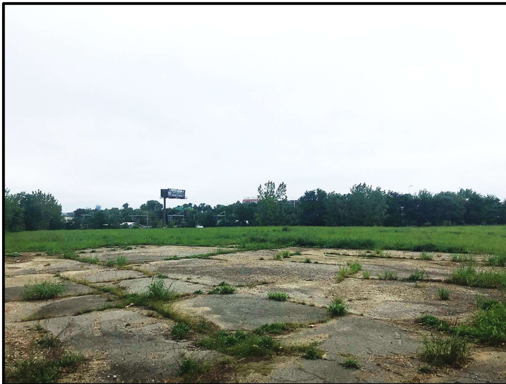
[2] View from Gate (Looking Northeast)
